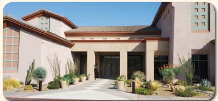
Delaware Room Entrance After
