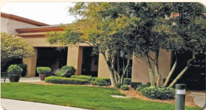
Delaware Room Entrance Before
