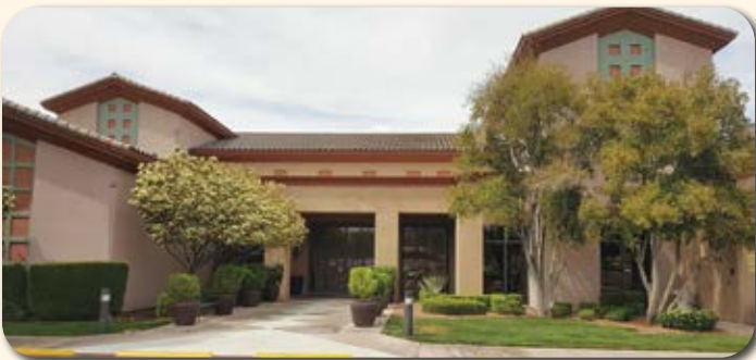
Delaware Room Entrance Before
