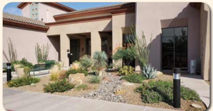
Delaware Room Entrance After
