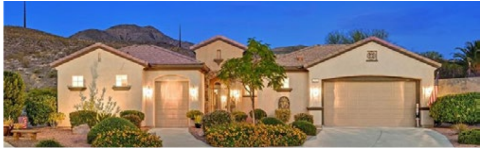
2153 Farmington Bay Ct., $999,500 2,746 sq.ft. 3-bd+1, 4-bath. Every window frames a picturesque view of Paradise! On a quiet cul-de-sac, this residence epitomizes high-end living. Embrace the beauty of nature in this unique Trenton model nestled in an exclusive enclave with gated courtyard with mountain views. Escape into your own private sanctuary.
